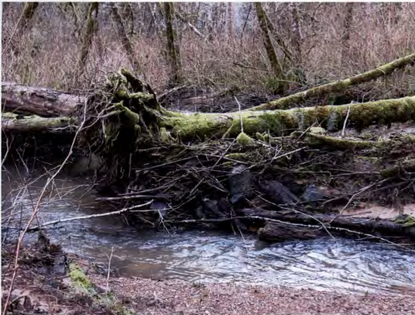
Figure 4. Site 6, looking downstream. This large alder with rootwad fell into the stream channel and was lodged into the site, further strengthening the structure.
