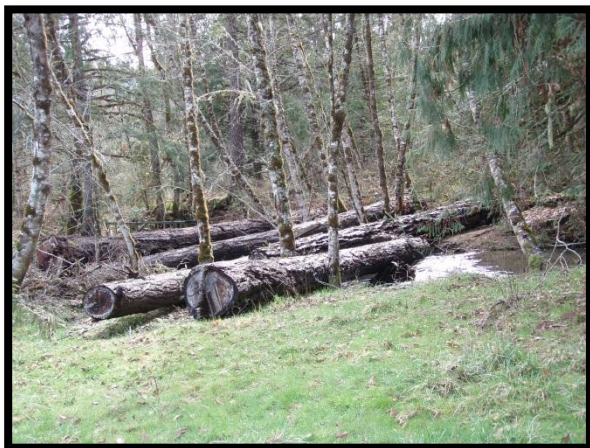
Photo 8: Completed instream log placement project upstream on Weaver Creek
