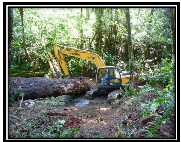
Large log being placed to improve salmonid habitat.
