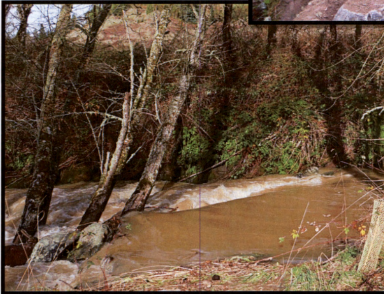
Photo #7 Days Creek Site 3 December 2012 during high flow event. This structure is slowing flow allowing substrate to drop out upstream as well as spreading the flow out to connect with the flood plane.
