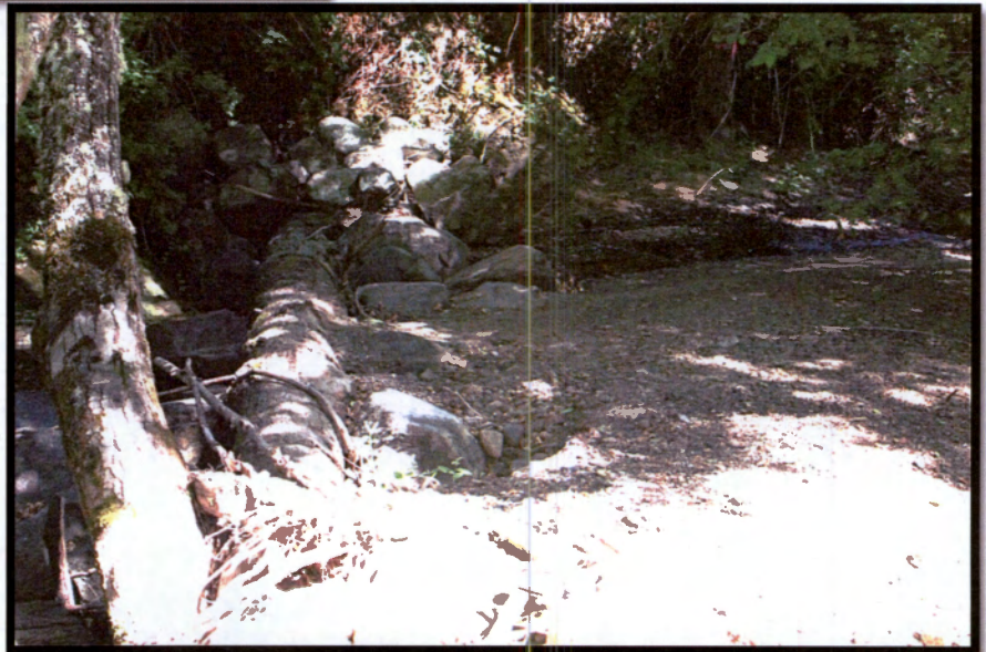
Photo #7 Days Creek Site 3 December 2012 during high flow event. This structure is slowing flow allowing substrate to drop out upstream as well as spreading the flow out to connect with the flood plane.
