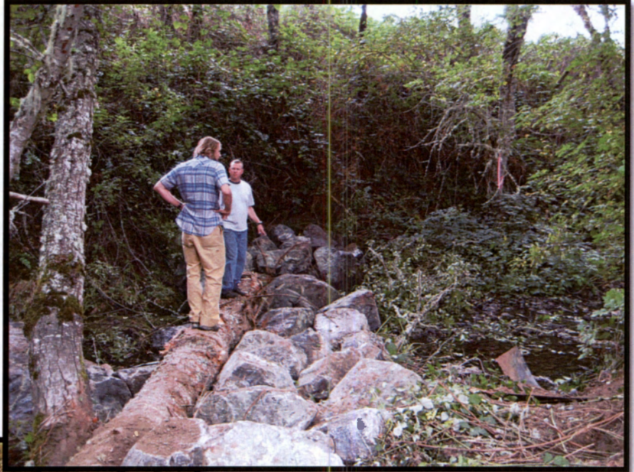
Photo #6 Days Creek Site 3 September 2010 Log and structure placement just after placement.
