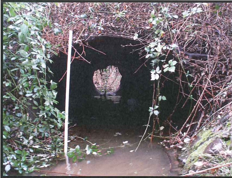
Briggs Culvert Inlet Pre-project 2009
