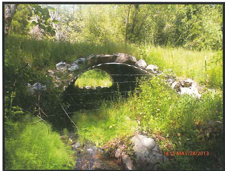
Briggs Culvert Outlet Post-project 2013
