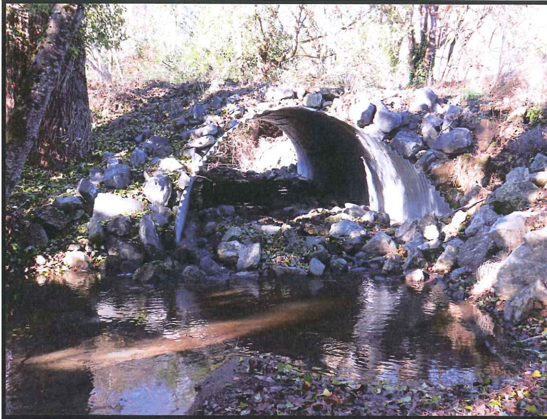
Battle Culvert Outlet Post- project 2012
