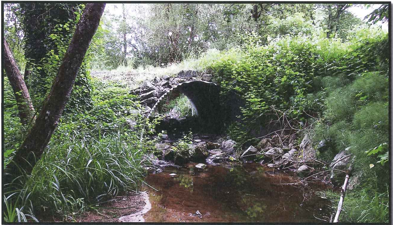
Battle Culvert Outlet Post-project June 2015. Culvert continues to function well.
