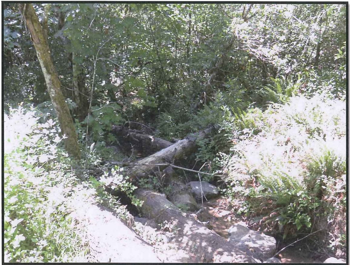
Site #12 Briggs Property Post- project June 2014
