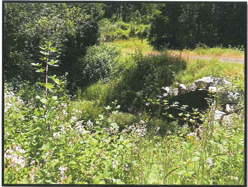
Briggs Culvert Inlet Post-project June 2014
