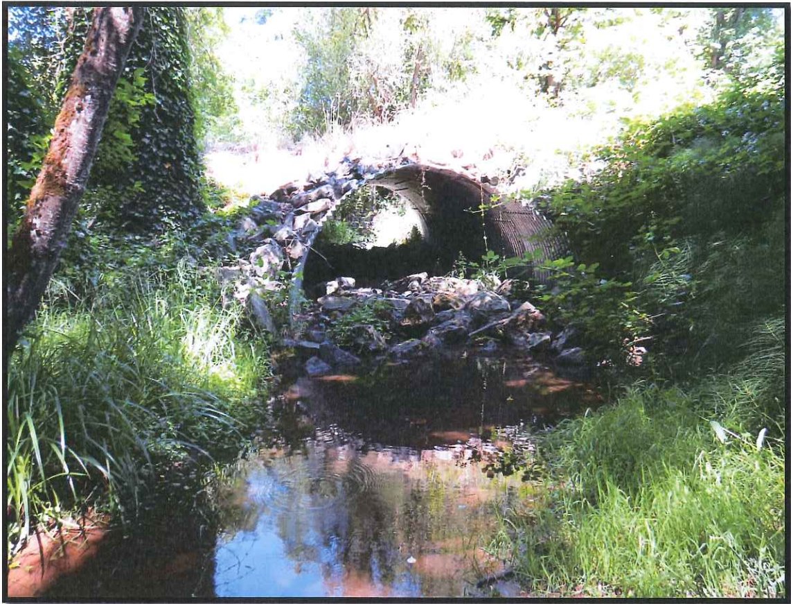
Battle Culvert Outlet Post-project June 2014
