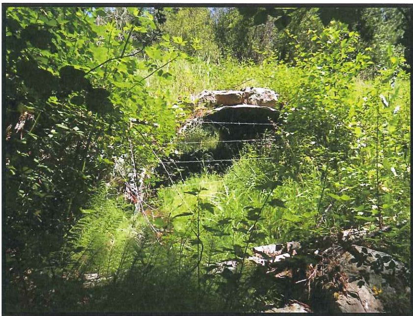
Briggs Culvert Outlet Post-project June 2014
