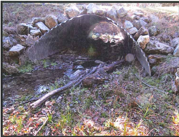
Briggs Culvert Outlet Post-project 2012
