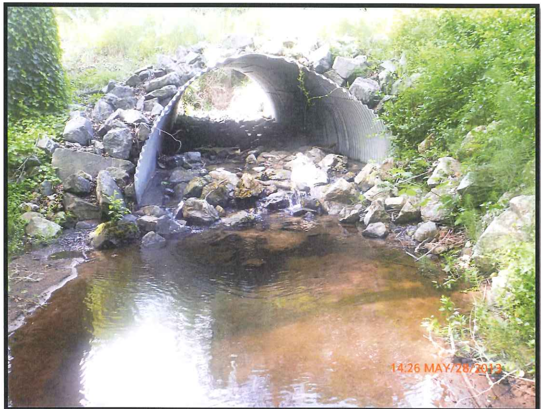
Battle Culvert Outlet Post-project 2013
