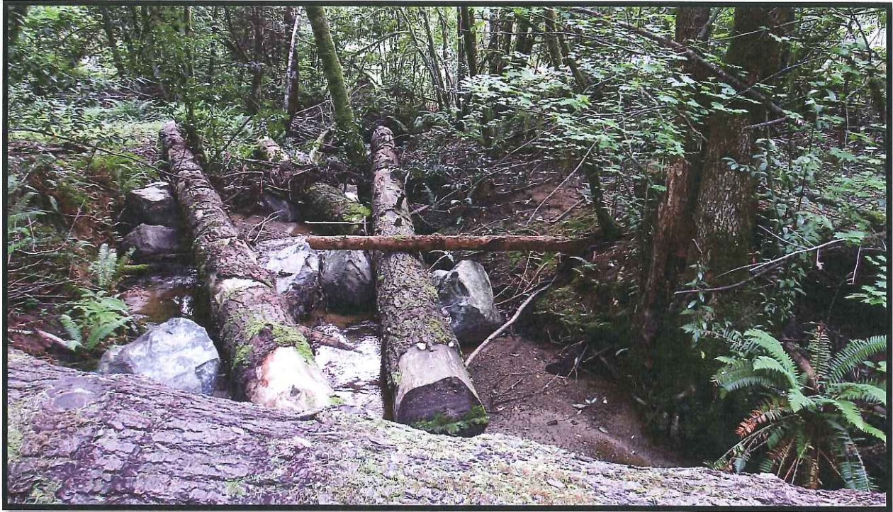
Site #21 Briggs Property Post-project June 2015. Sand deposits are seen far up into the floodplain after the Dec. 21 st , 2014 storm came through. This high water event was estimated to be a 20 year return interval event. The logs held firm in this flow and complexity continues to increase with increased gravel and sand deposition.
