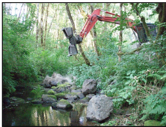
Above: Contractor Gary Rundell placing boulders in Little Tom Folley Creek
