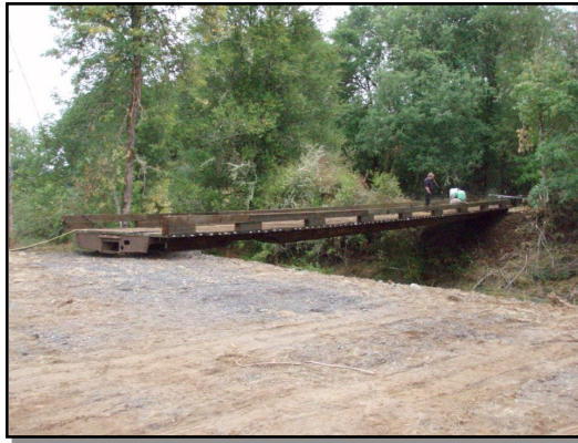
Above: Railcar Bridge installed over Olalla Creek
