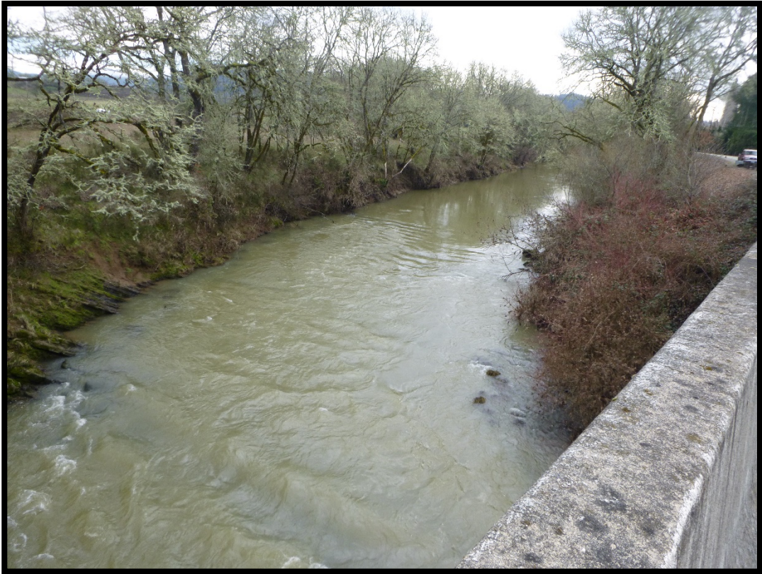
Photo 1. Calapooya Creek below at Garden Valley Road Bridge 2/14/17
