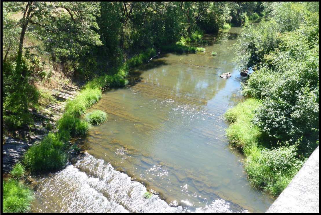
Photo 2. Calapooya Creek below at Garden Valley Road Bridge 7/14/2016
