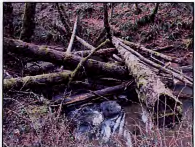
Figure 1d. Site 1, looking downstream. Post-Project 2/15/2016
