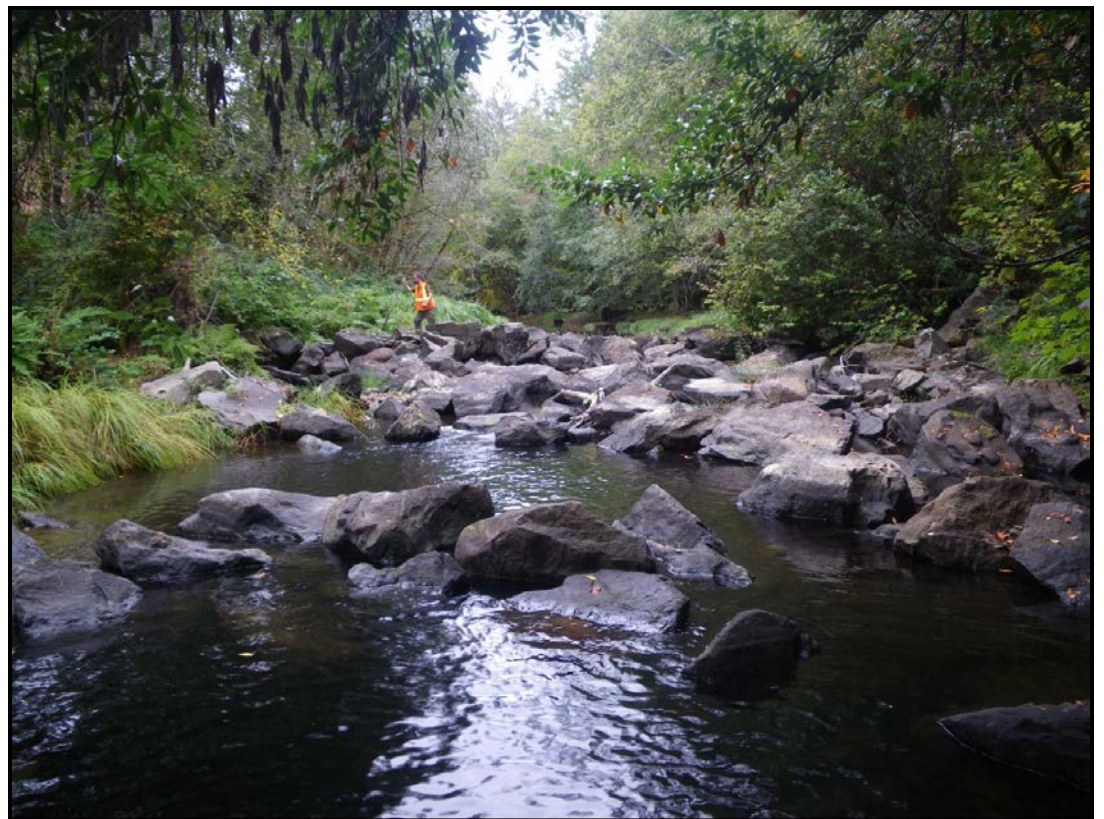
Photo #30: Weir #9 from downstream looking upstream 10/14/12
