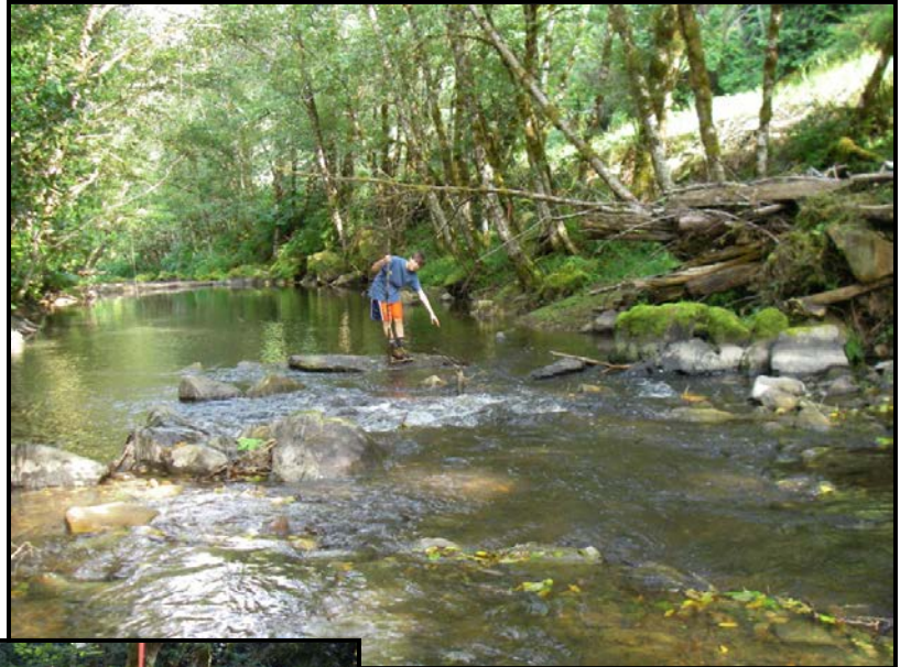
Photo #33: 7/27/09 Weir#10 and gravel placement day of construction N43 26.117 W123 35.572 Weir Length 82' Active Channel Width 34' 146 Boulders 100 cu.yd. - 6' minus unsorted unwashed gravel
