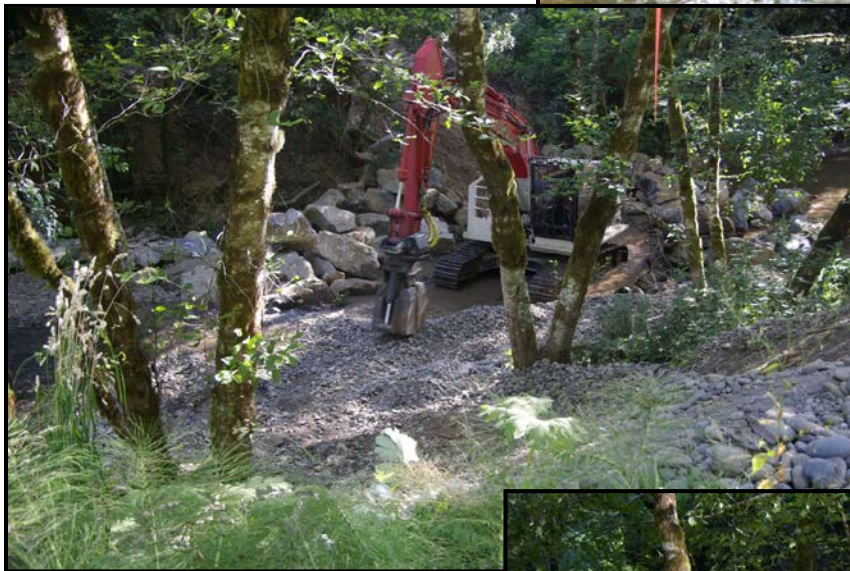
Photo #33: 7/27/09 Weir#10 and gravel placement day of construction N43 26.117 W123 35.572 Weir Length 82' Active Channel Width 34' 146 Boulders 100 cu.yd. - 6' minus unsorted unwashed gravel
