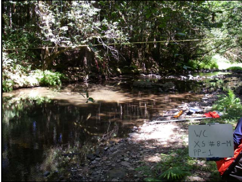
Photo 3: 7/6/2009 Proposed site Weir #8 Looking downstream at weir
