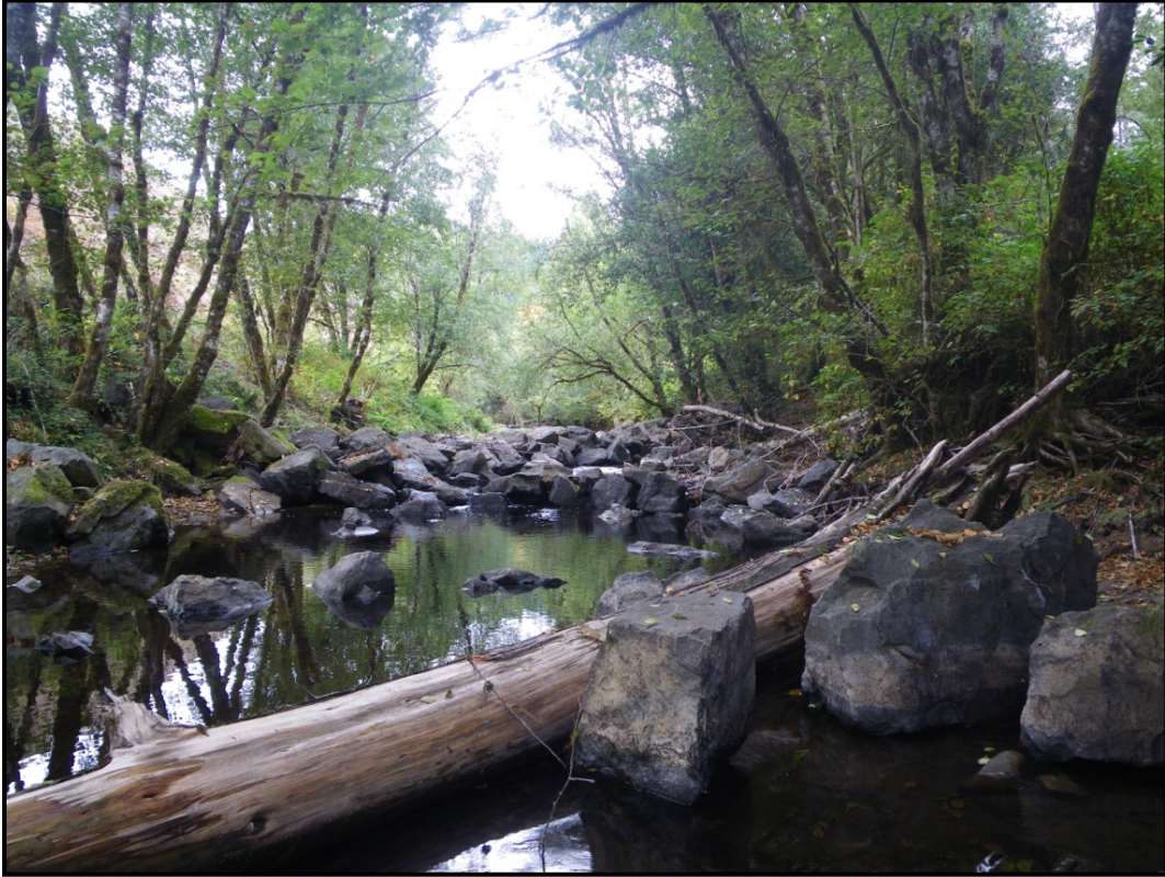
Photo #39: Weir #10 from downstream looking upstream 10/14/2012
