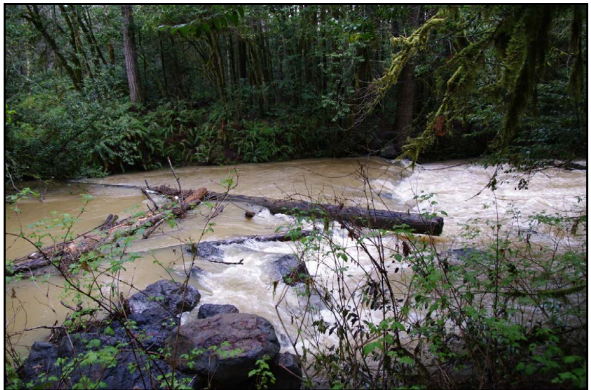
Photo 8: Weir #8 3/31/2010 Following a major storm event
