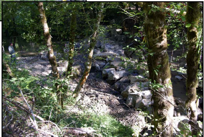
Photo #33: 7/27/09 Weir#10 and gravel placement day of construction N43 26.117 W123 35.572 Weir Length 82' Active Channel Width 34' 146 Boulders 100 cu.yd. - 6' minus unsorted unwashed gravel
