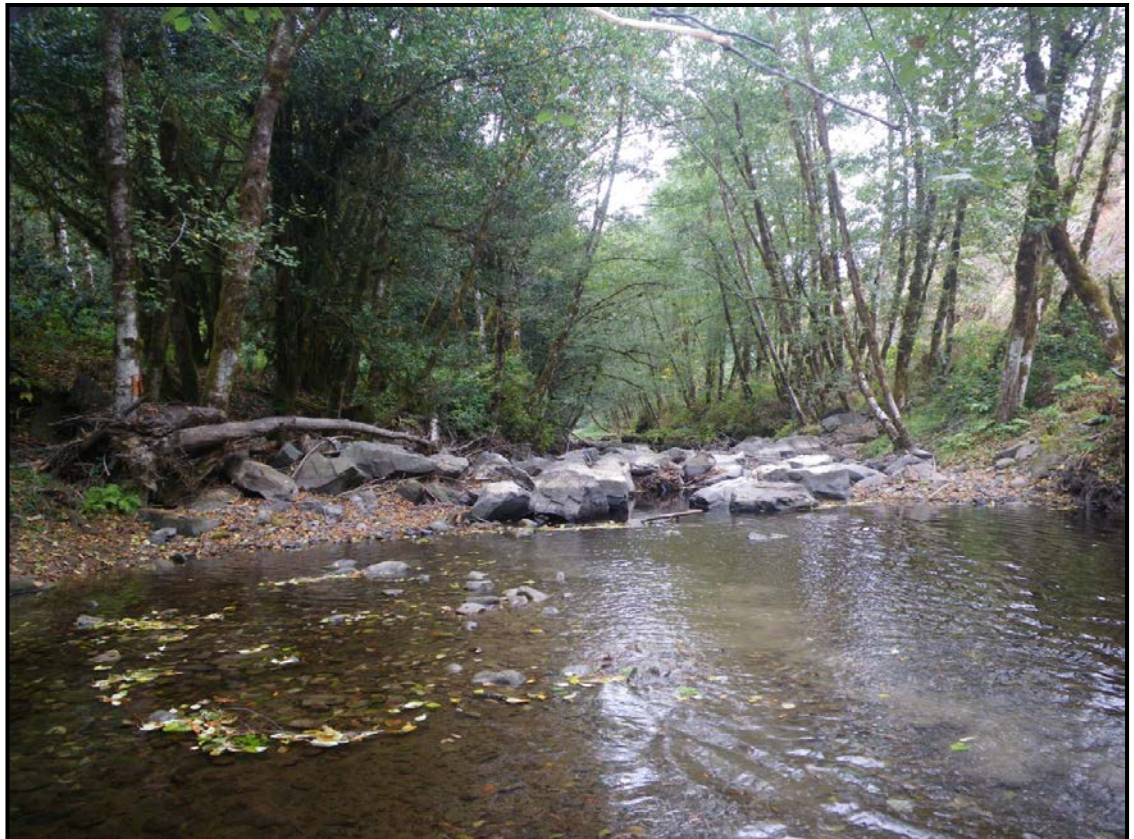
Photo #40: Weir #10 from upstream looking downstream 10/14/2012
